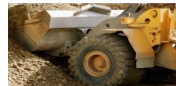
Land reclamation / Earthworks
